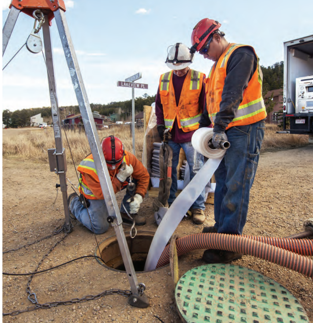
Tom Spiegel, Allen Hamm and Erik Gomez (from left) install slip foil to the bottom of the sewer line to protect and allow for easy installation of the fiberglass reinforced liner.
